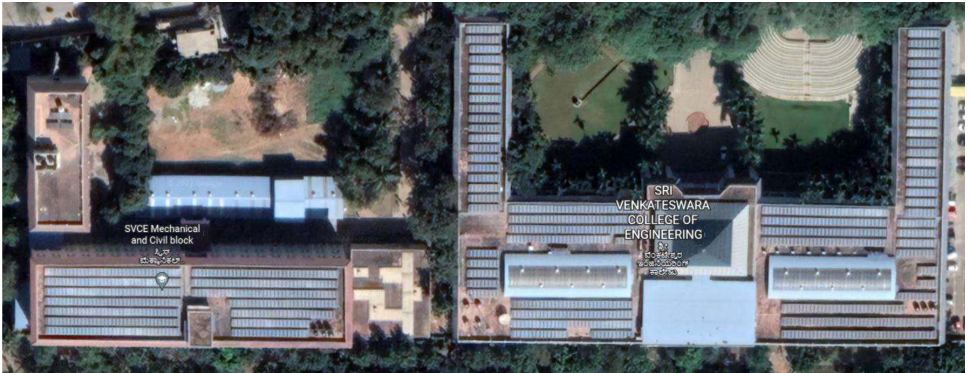
Google map view of rooftop solar panel at Sri Venkateshvara College of Engineering, Bengaluru-562157
